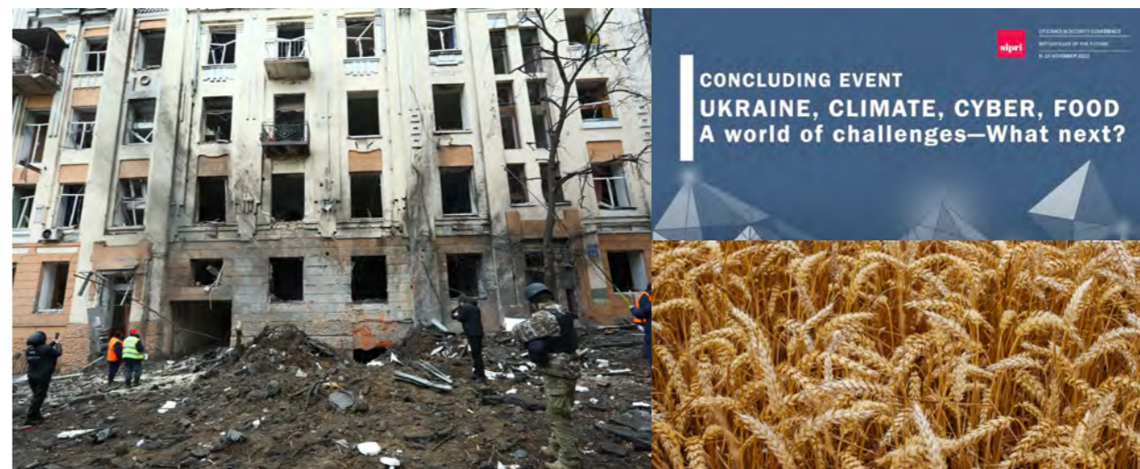
Left: A damaged building in Kharkiv, Ukraine, after Russian rocket strikes.
