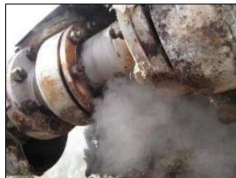
Deficiency in steam line
