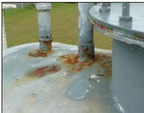
Corrosion of fuel tank for equipment facility
