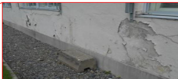
Cracks in the wall
