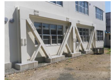
Seismic retrofitting of barracks (conceptual image)
